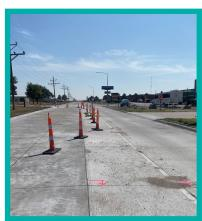
Country Club Drive in Colby is a main road connector between US-24 and I-70. To help meet demand, construction is underway from E College Drive north to the first set of railroad tracks. The project is widening the roadway to accommodate three 12-foot lanes, including a two-way left turn lane.
